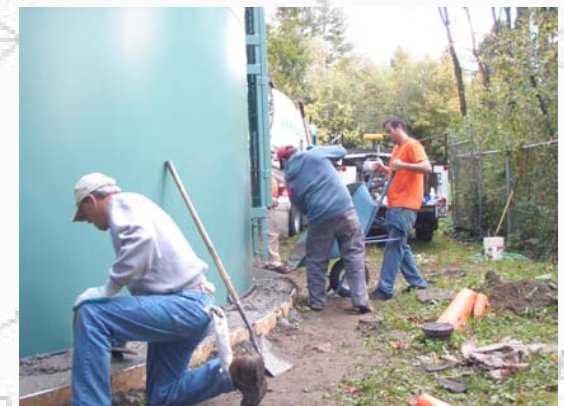
District Staff installing corrosion protection anode footing on reservoir
