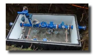
Over the last several years customers in our Beach Zone experienced pressure fluctuations due to intermittent failure of an aging pressure reducing valve station.
