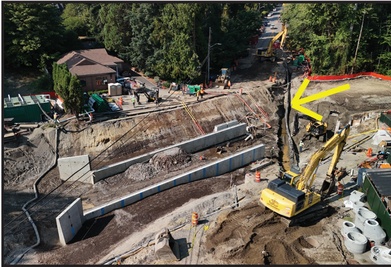
Aerial view from September
