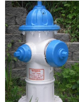
Lake Forest Park Water District Hydrant
