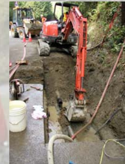
← Contractor installing new watermain on 45 th Pl.
