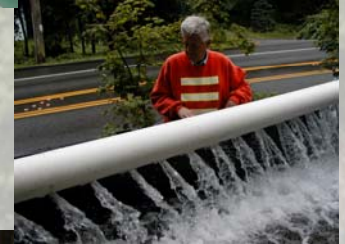
Roy Blackwell monitors watermain flushing discharge pipe header and stilling tank →
